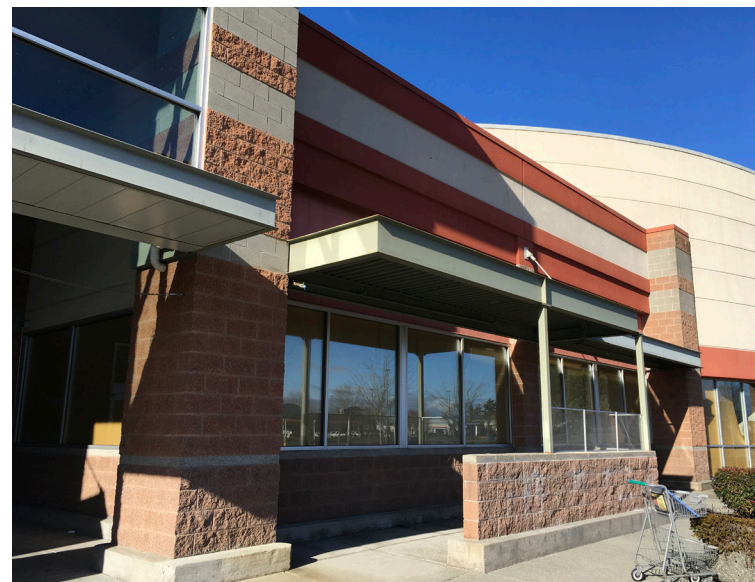
Location B Cart Area with Pony Wall
