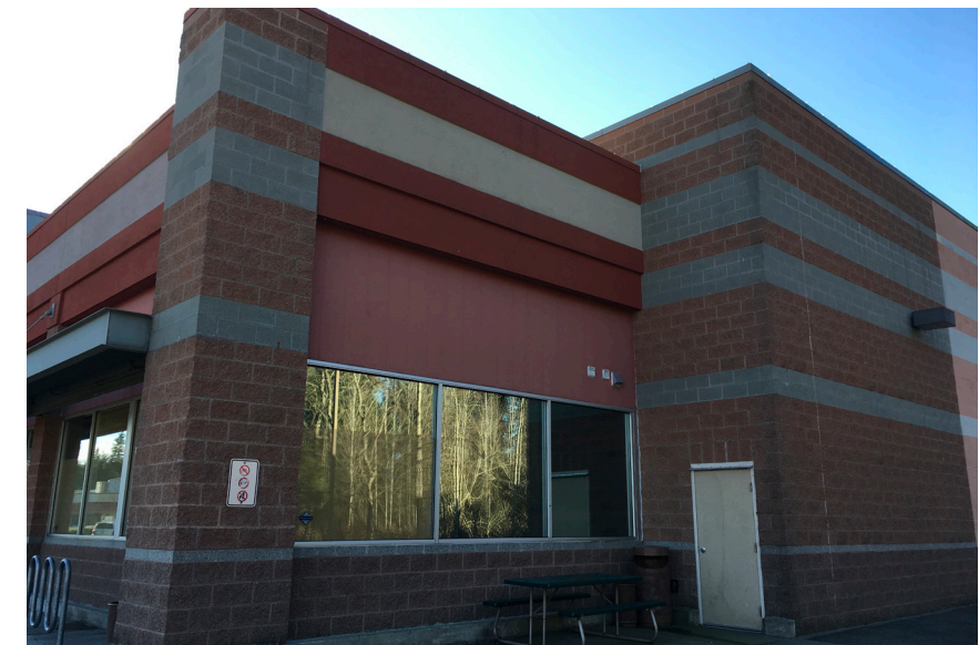
Location D Side of Building Front
